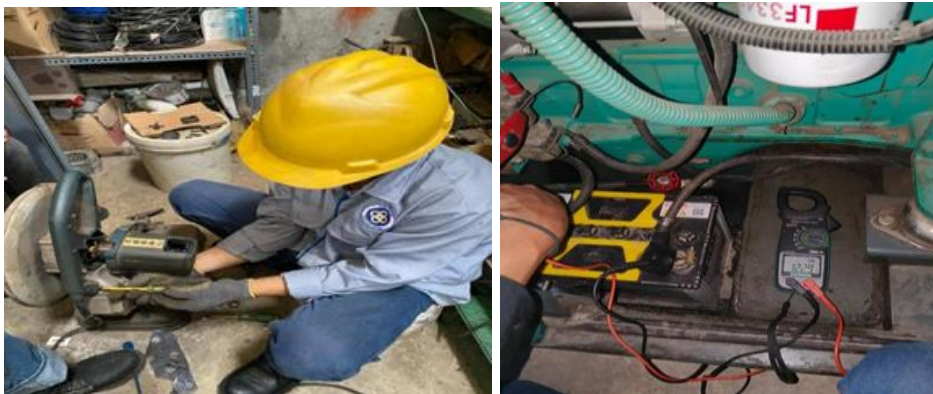
Gambar 1. Maintenance Cutting Wheel dan Pengukuran Daya Aki Genset
